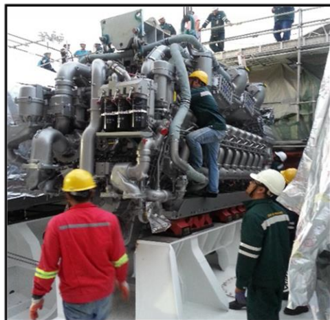
Main Engine Installation
