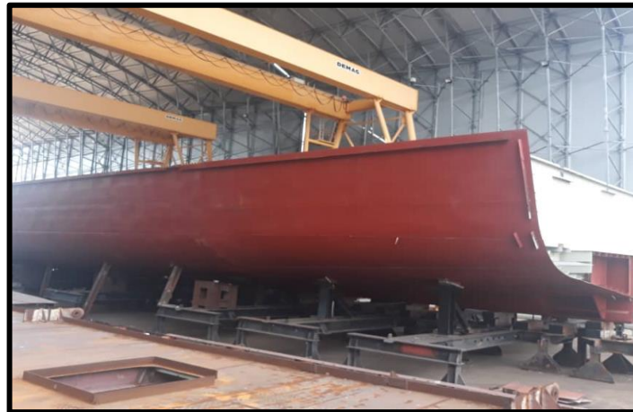
Main block erection
