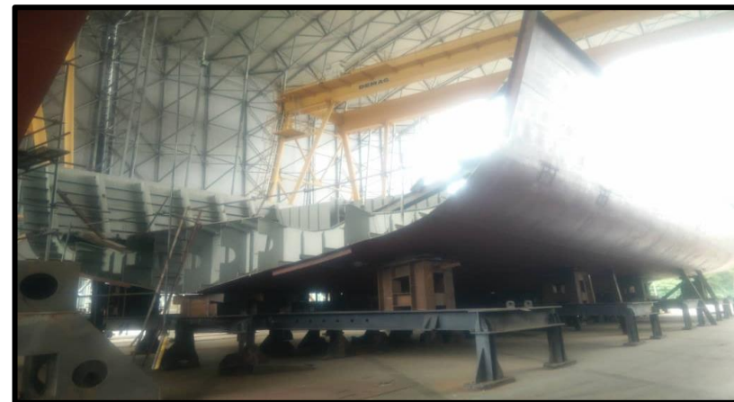
Main block erection
