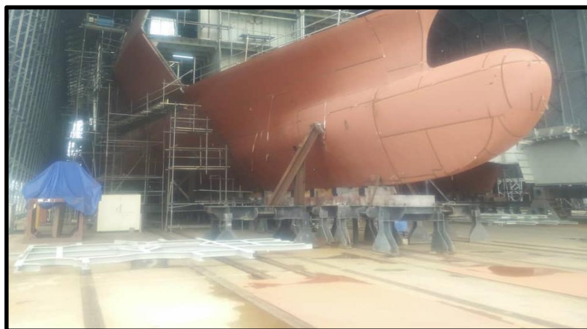
Joined hull (forward section)
