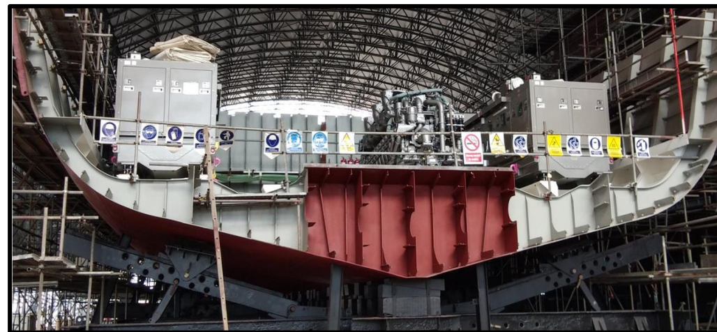
Main equipment installed before block joining
