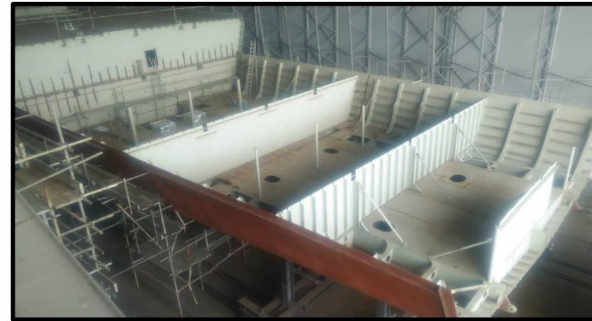
Main block erection
