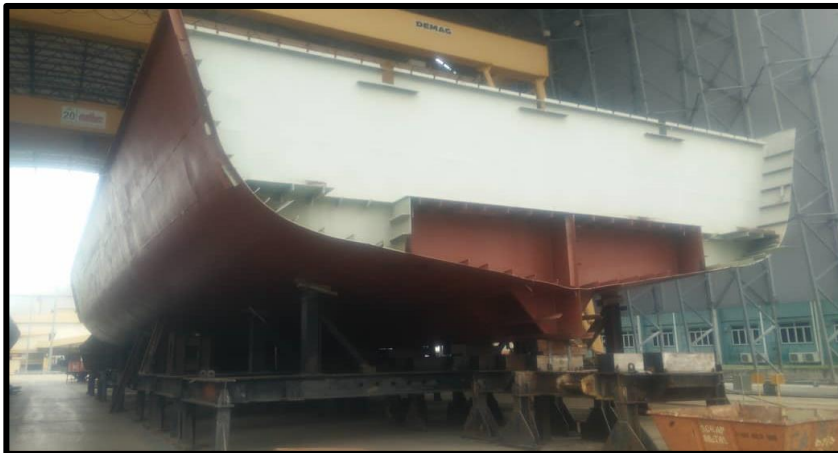
Main block erection
